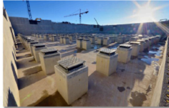
In 2013, work will begin on the basement floor which will be supported on the columns and seismic bearings.
