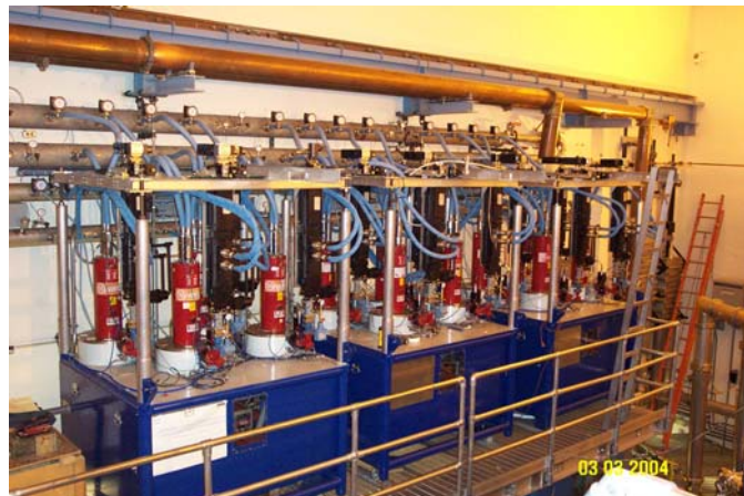
Figure 3.1.8: Klystron mezzanine showing klystrons and the circulators now undergoing high power testing.
