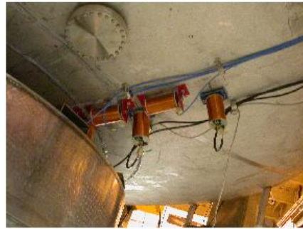
Figure 3-7: Actual pictures of the B_p coils and flux loops as installed at the top (top right), side (left), and bottom (bottom right) of the vessel.
