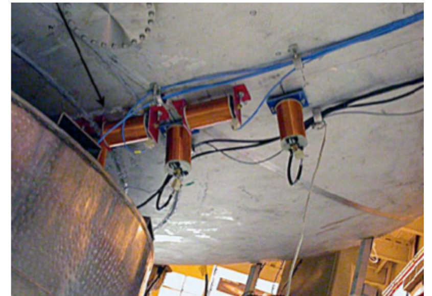
Poloidal field coils
