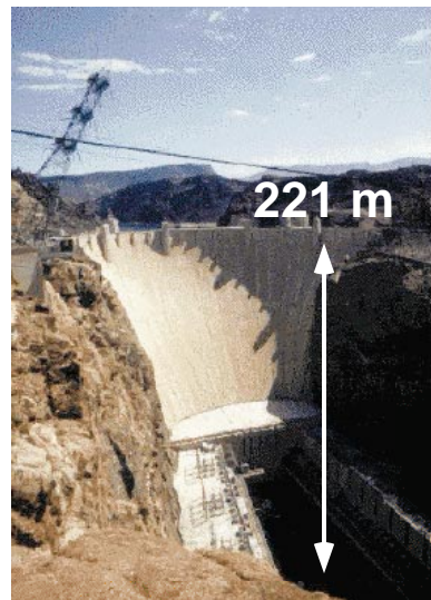
Hoover Dam, located on the Colorado River in southeastern Nevada, was opened in 1936. The impounded waters formed Lake Mead, 185-km-long, one of largest artificial lakes in the world. The dam, 221 m high, is used for flood control, irrigation, and power.
