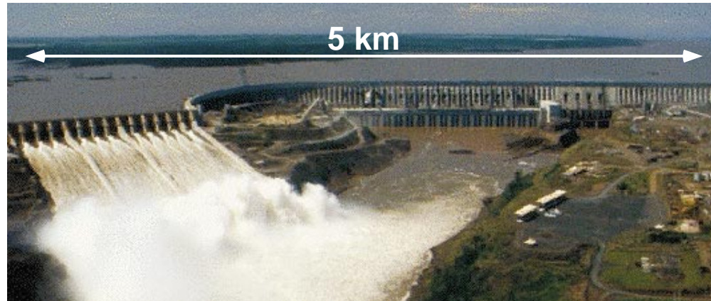
The Itaipu Dam, completed in 1982 on the Parana River between Brazil and Paraguay, will eventually generate 12,600 MW, making it the largest power complex on Earth. The Itaipu Dam is 8 km long and cost $20B.
