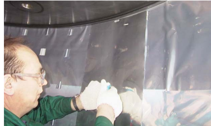
Installation of monocrystalline Al coated SS sheets
