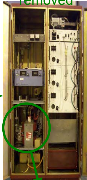
Cabinet with doors removed
